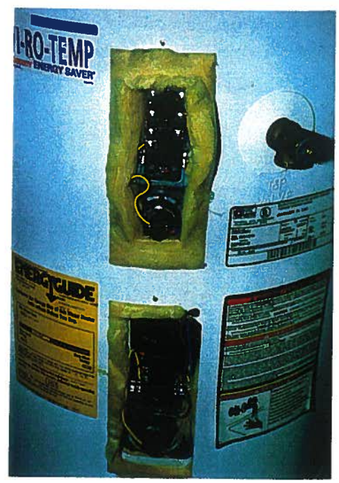
PHOTO 1—“Low boy” electric water heater with side covers removed showing thermostats, wiring and heating element connections.
