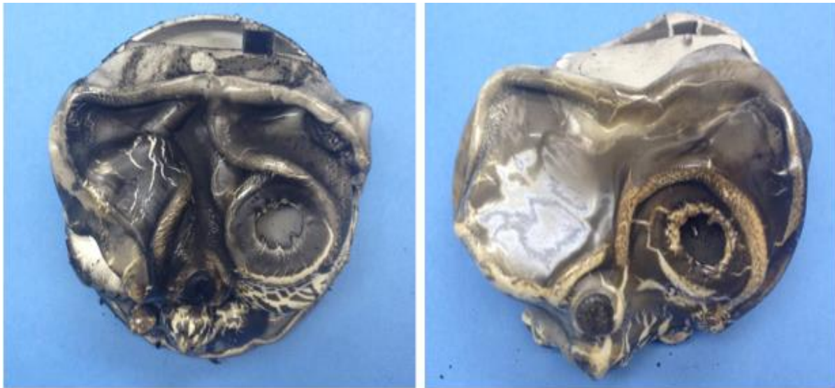
Figure 6 – Smoke detectors that were damaged during the fire.
